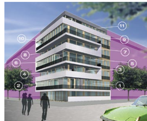
>> Sc11 Baugruppe, Schönholzer Straße 11, Berlin
